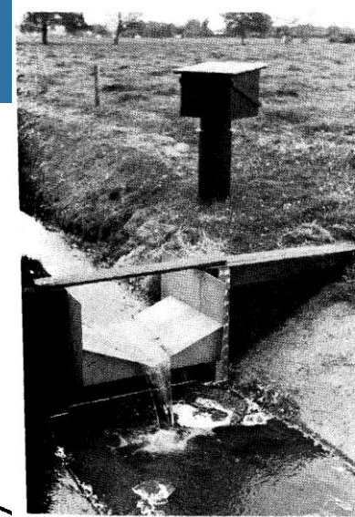
Photo 2 Triangular broad-crested weir
