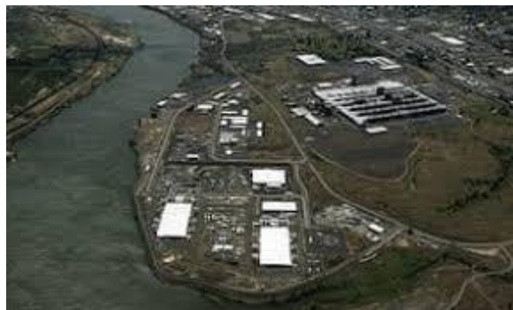
FIGURE 1.1 The Google Dalles, Oregon, datacenter shown in Google Earth is an industrial-sized information technology utility.
