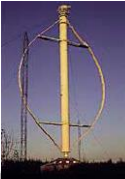
Vertical axis Turbine
