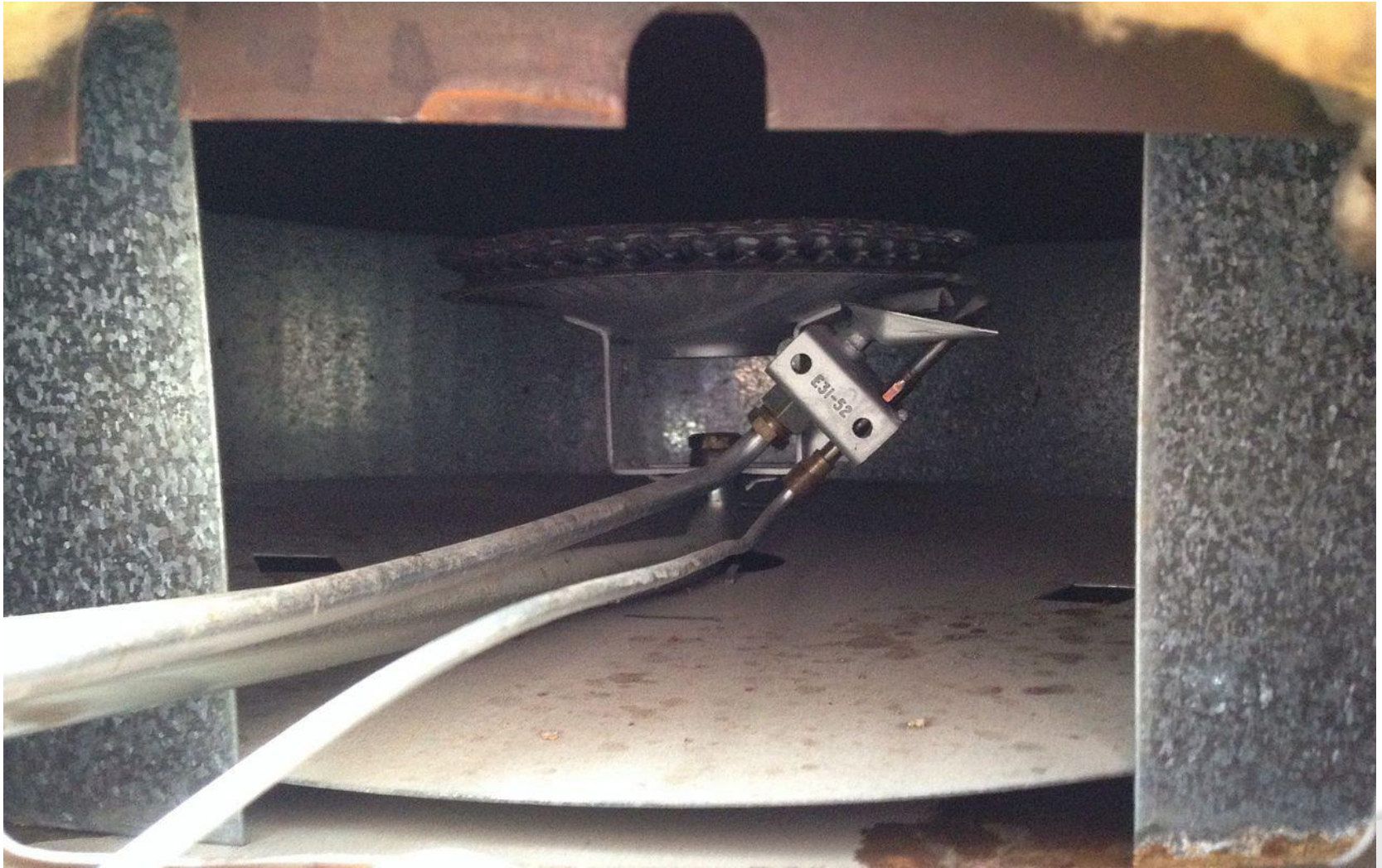
Thermocouple (the right most tube) inside the burner
