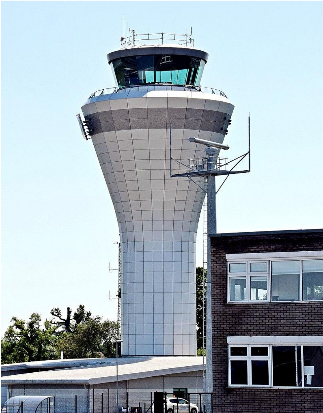
Fig 5.4 Air traffic control
