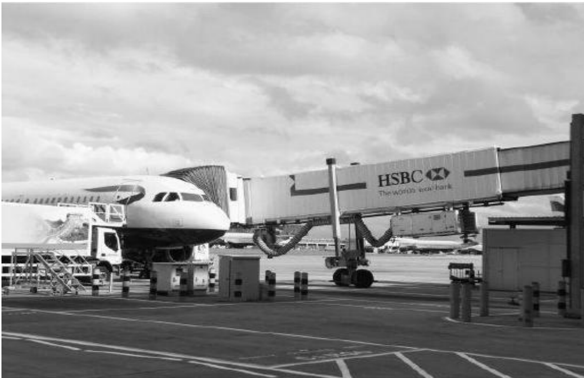
Fig 2.5 Elevating passenger air bridge
