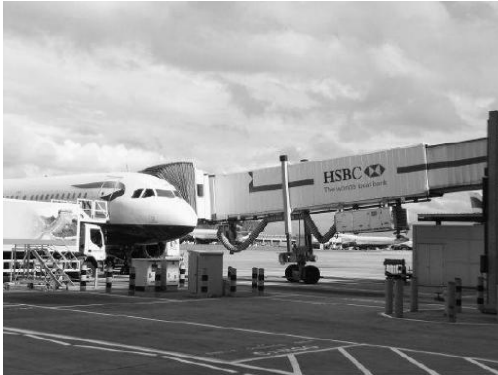
Fig.3.3 Elevating passenger air bridge
