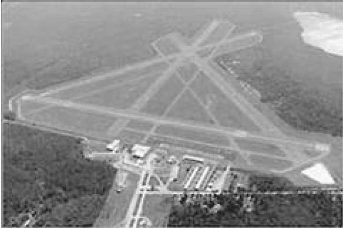
Fig.1.10 Flagler County Airport in Bunnell
