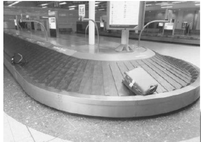
(a) Flatbed reclaim. (b) Inclined reclaim
