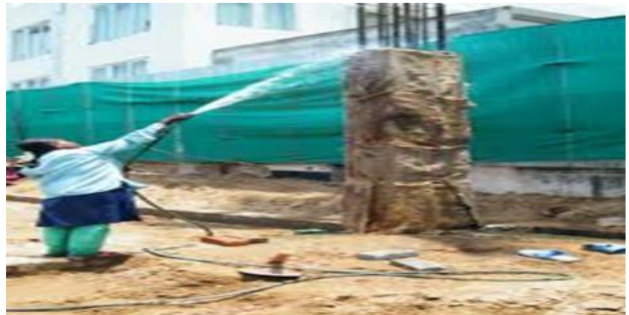
Fig: Water curing
