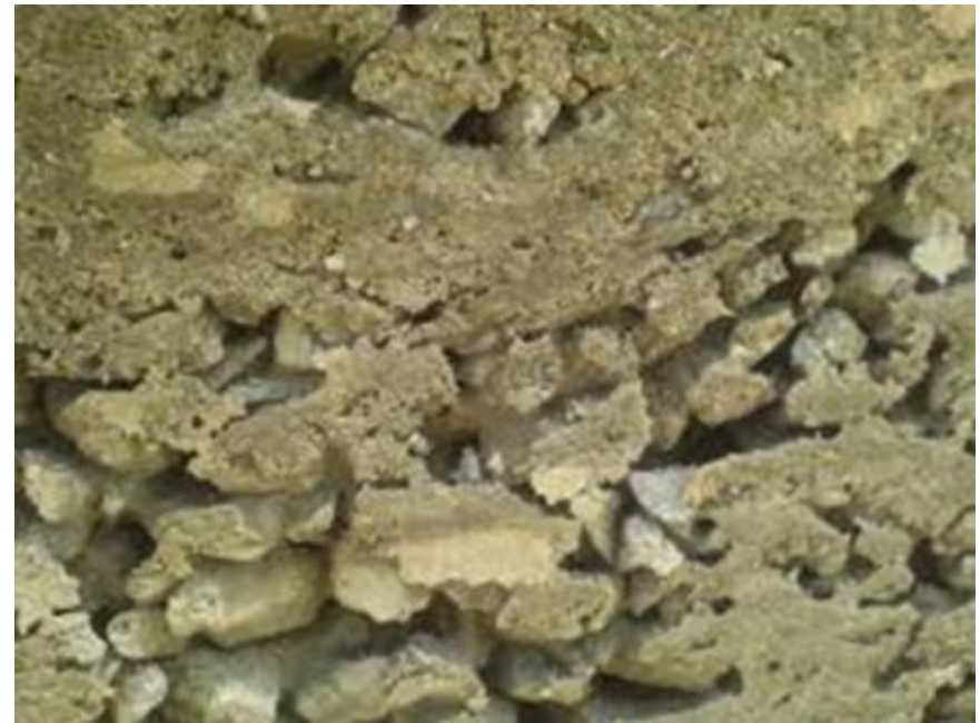
Fig: Segregation in concrete
