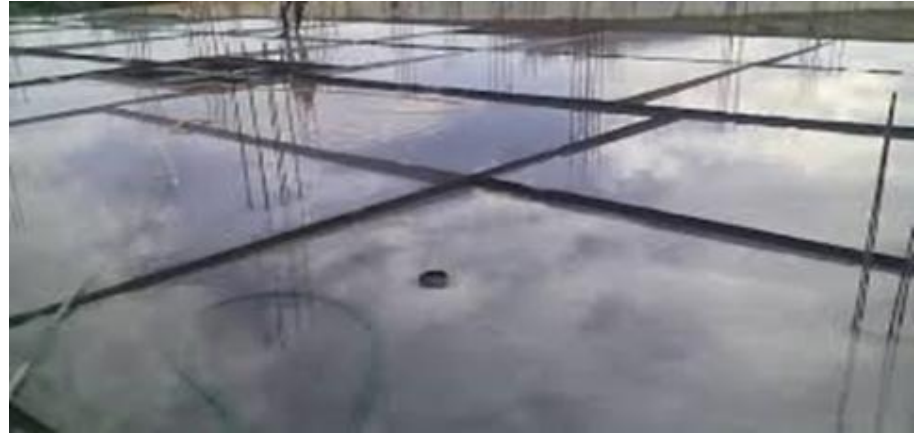
Fig: Water curing
