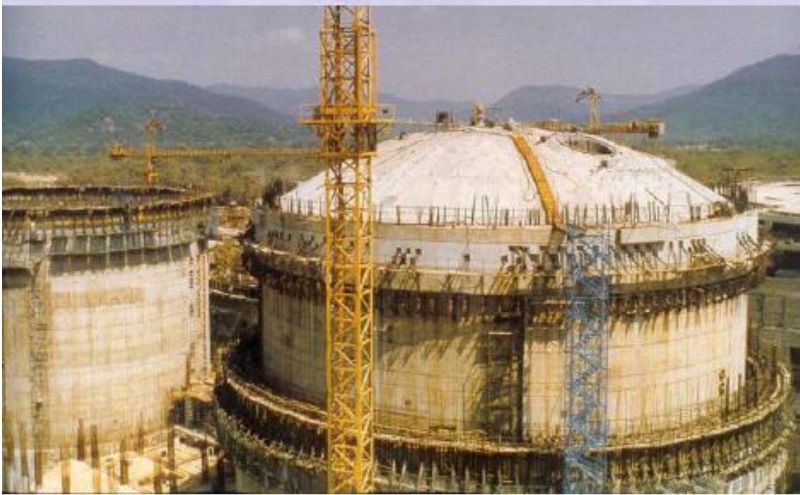
Figure: pre stressing of circular tank
