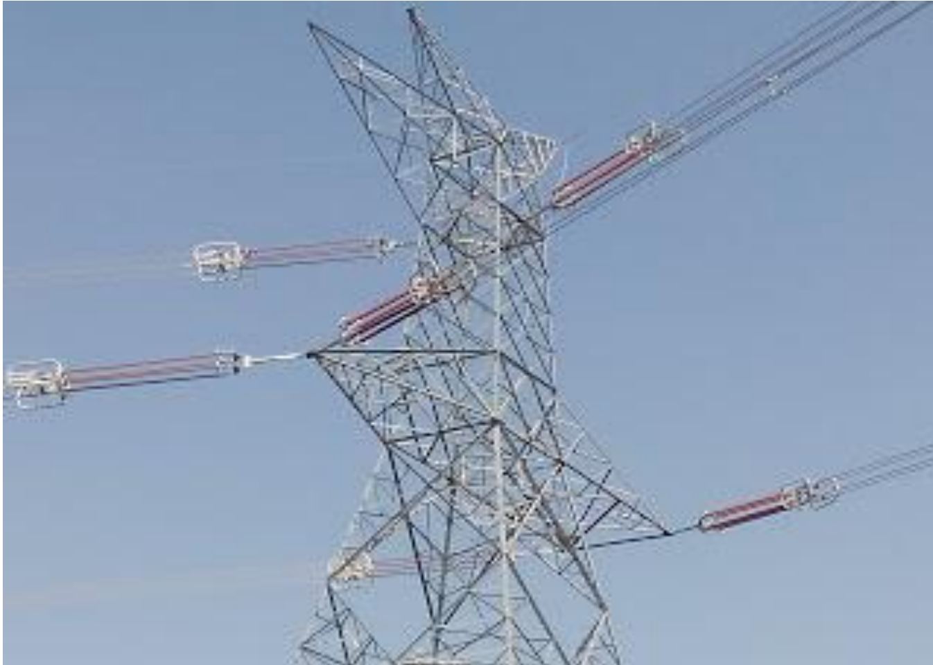
Fig.9: 765 kV transmission line in India with 4 sub-conductors per phase (Quadruplex bundle).
