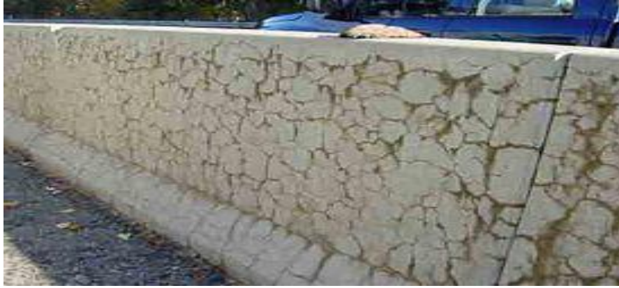
Typical effect of Alkali-Aggregate Reaction
