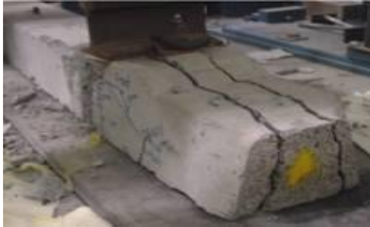
Fig. 2 Load induced deterioration
