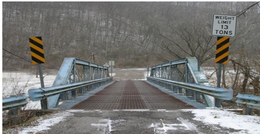
...y metal truss
