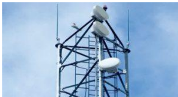
Microwave Transmission Node
