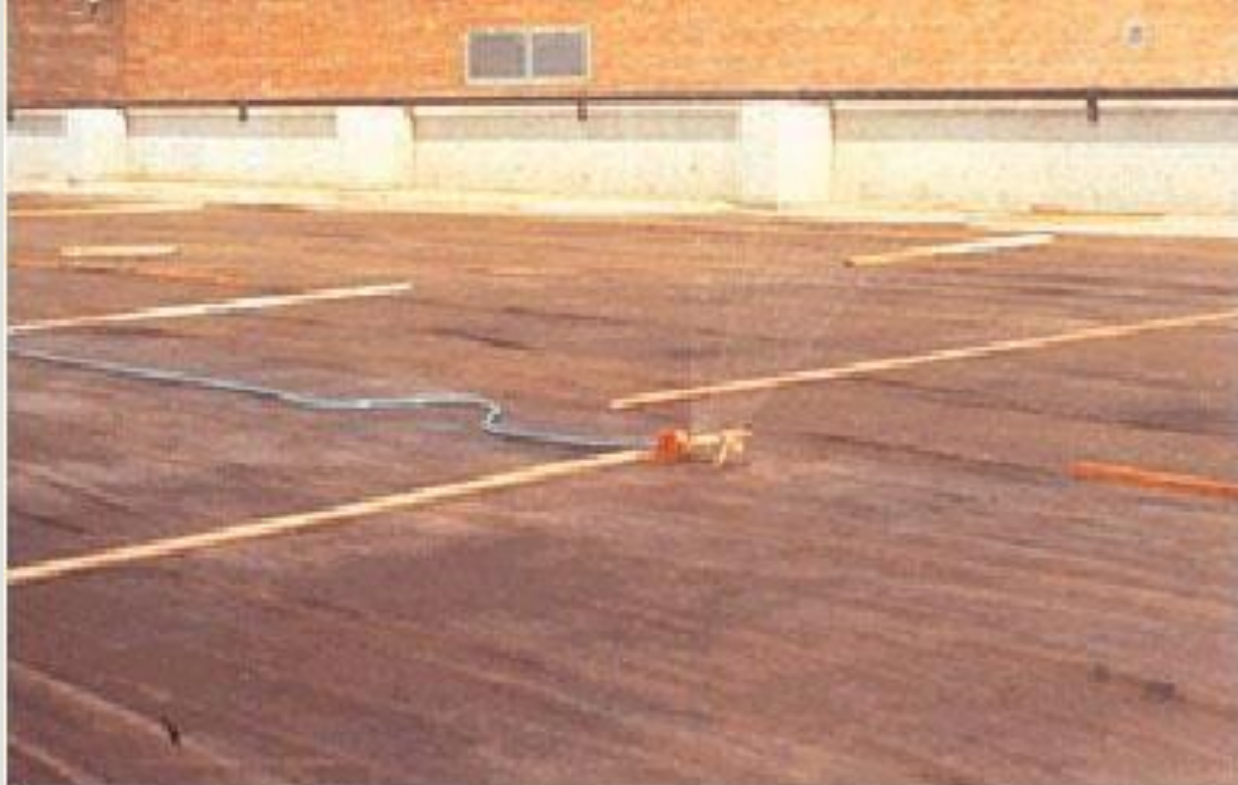
Fig. 12-5. Lawn sprinklers saturating burlap with water keep the concrete continuously moist. Intermittent sprinkling is acceptable if no drying of the concrete surface occurs. (50177)
