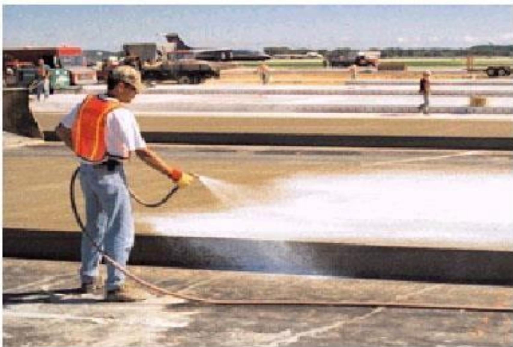
Fig. 12-8. Liquid membrane-forming curing compounds should be applied immediately following final finishing, with uniform and adequate coverage over the entire surface and edges for effective, extended curing of concrete. (69975)
