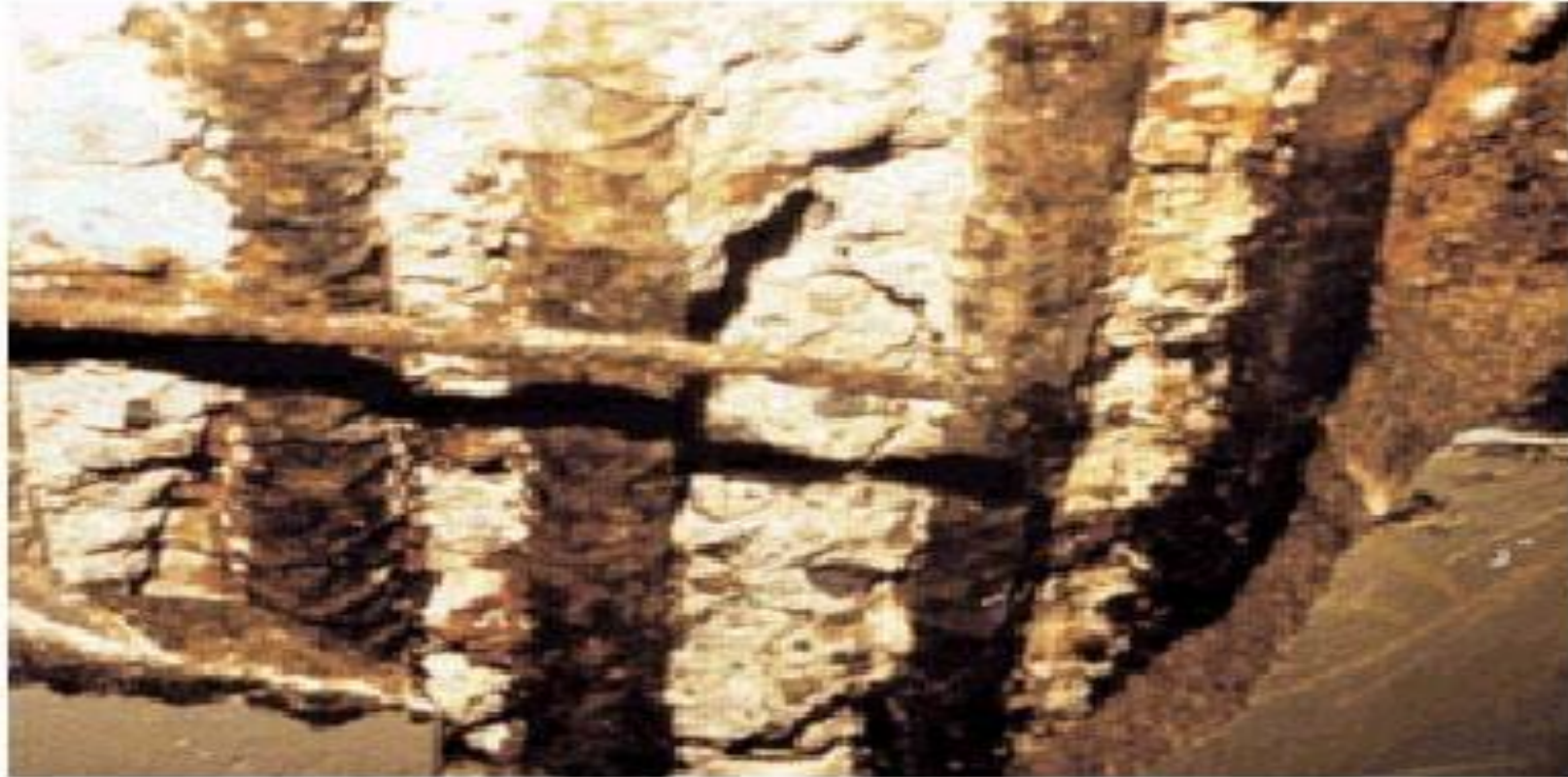
Fig. 6-16. The damage to this concrete parking structure resulted from chloride-induced corrosion of steel reinforcement. (50051)
