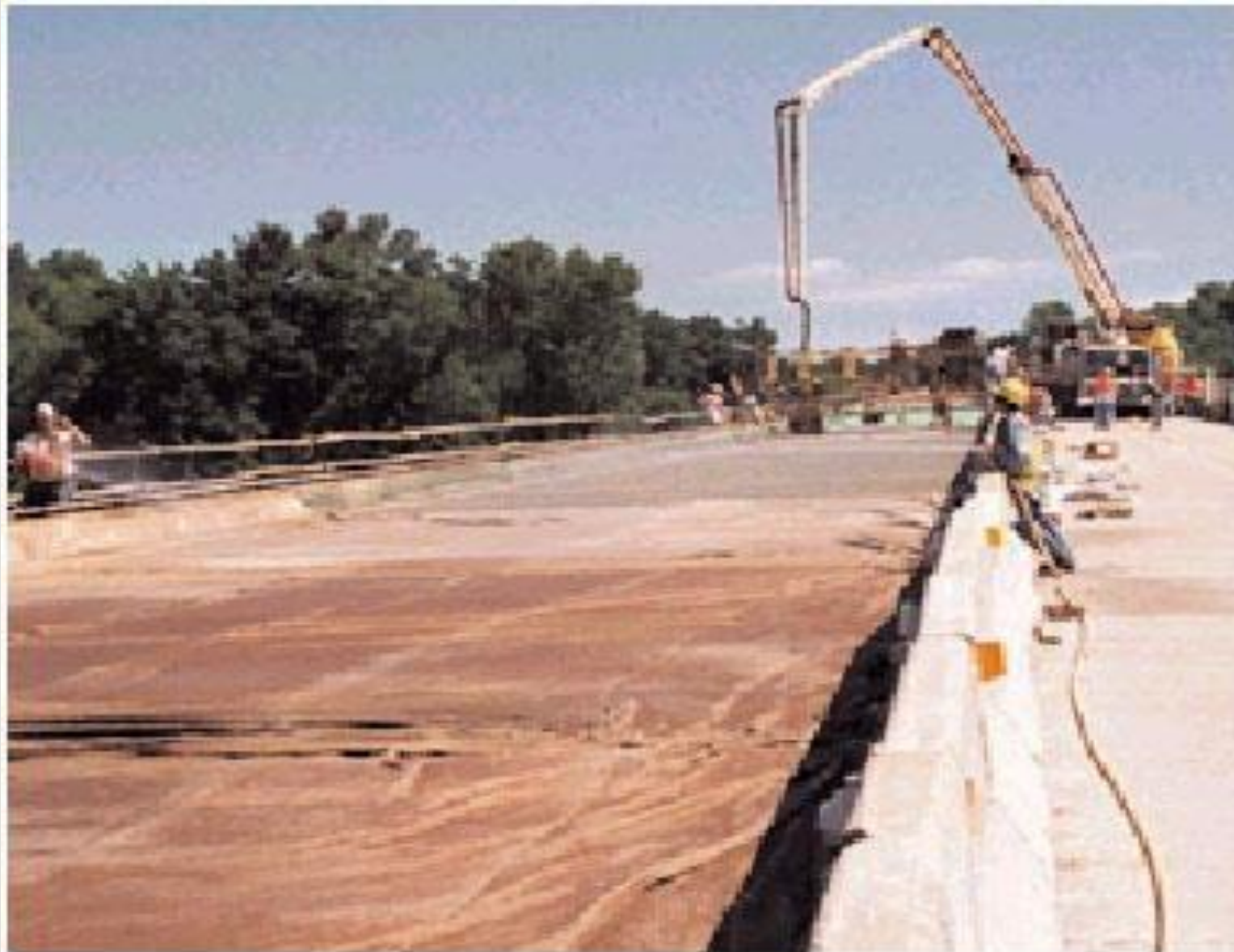
Fig. 12-1. Curing should begin as soon as the concrete hardens sufficiently to prevent marring or erosion of the surface. Burlap sprayed with water is an effective method for moist curing. (69973)
