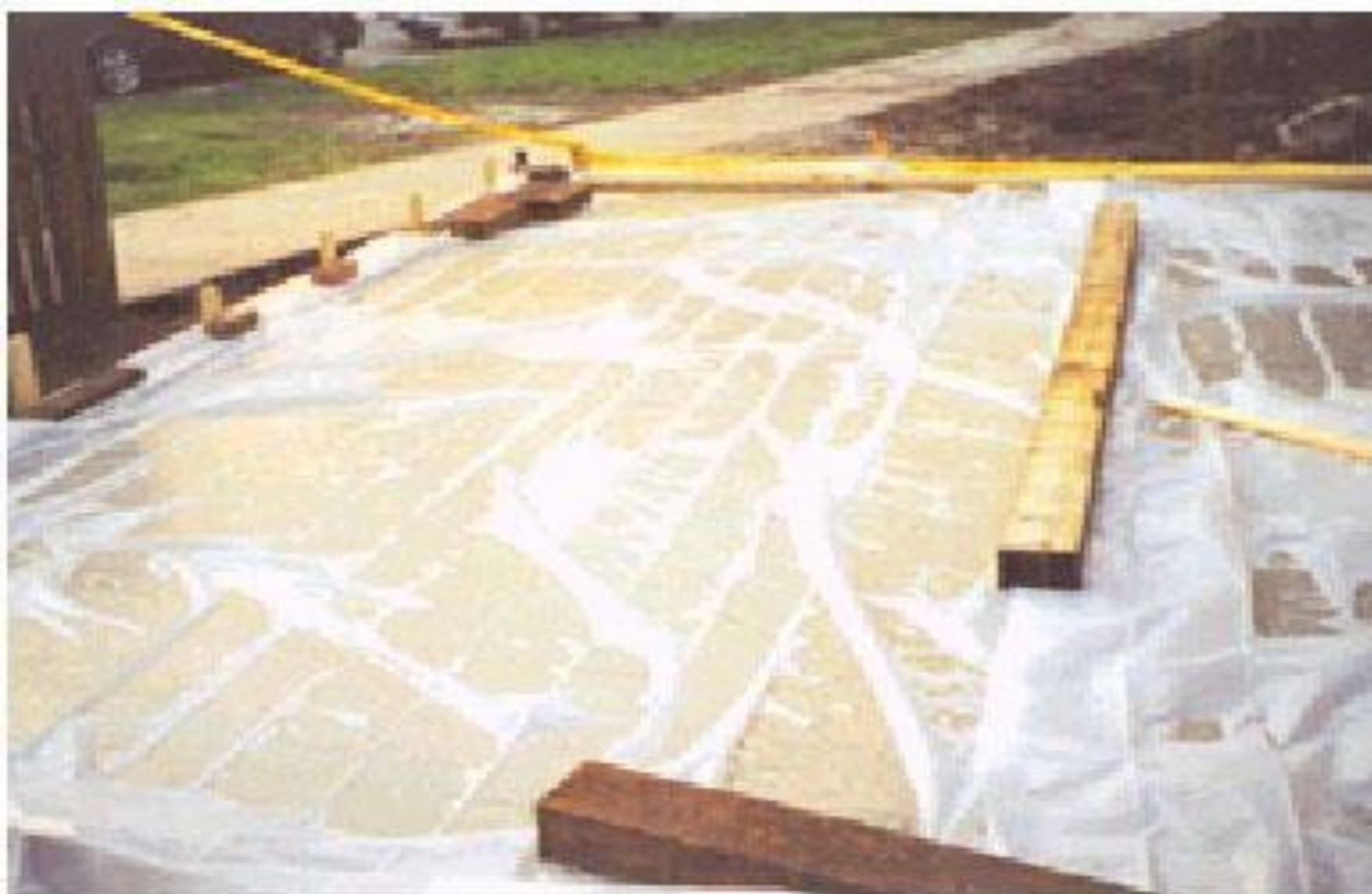
Fig. 12-7. Polyethylene film is an effective moisture barrier for curing concrete and easily applied to complex as well as simple shapes. To minimize discolouration, the film should be kept as flat as possible on the concrete surface. (70014)
