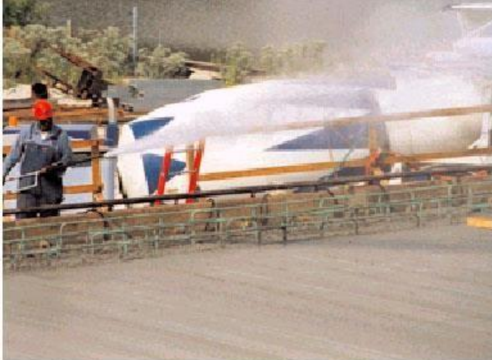
Fig. 12-4. Fogging minimizes moisture loss during and after placing and finishing of concrete. (69974)
