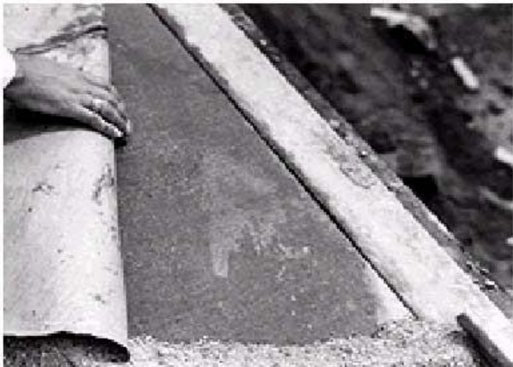
Fig.12-6. Impervious curing paper is an efficient means of curing horizontal surfaces. (69994)
