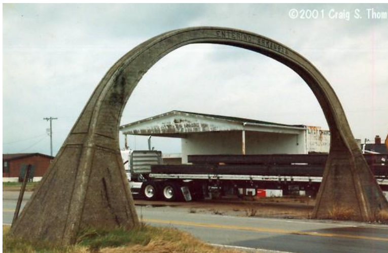
CONCRETE-takes more compression
