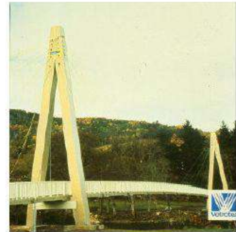
GFRP pedestrian bridge:
