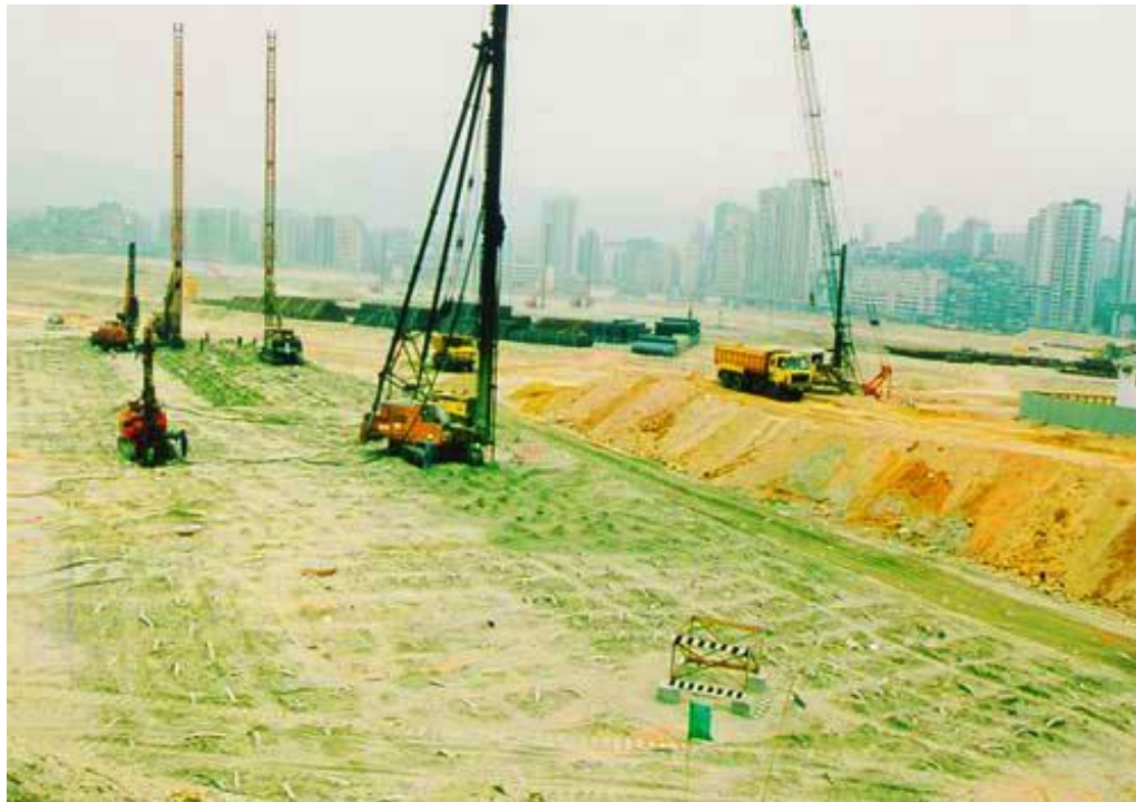
Installation of PVDs
