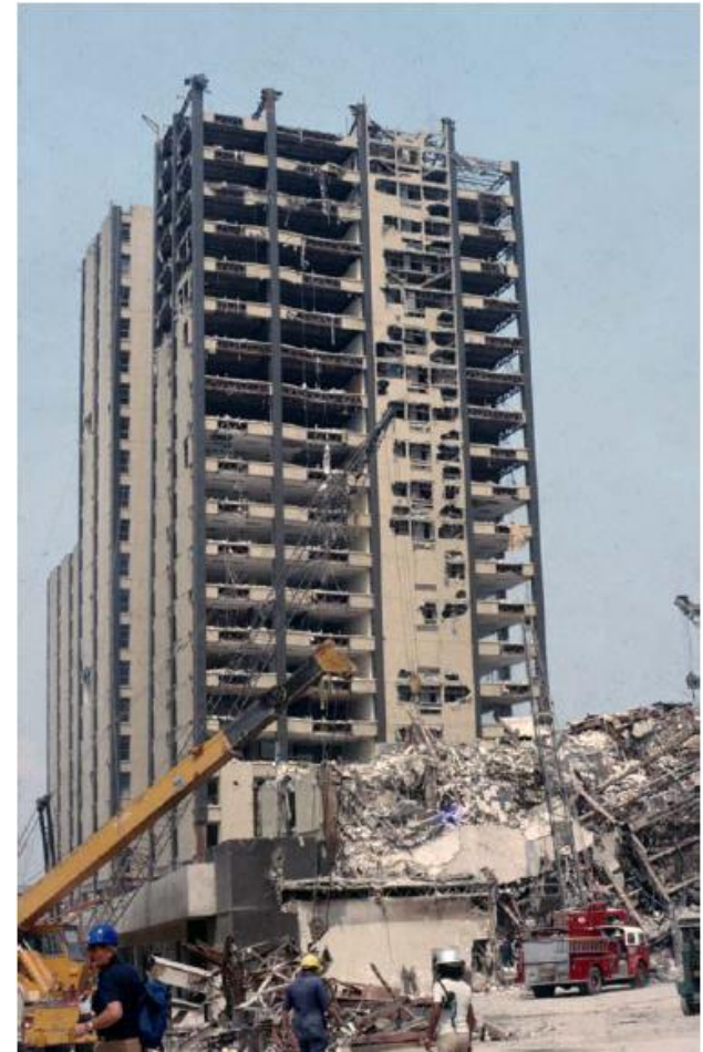
Damage to a Steel building in Mexico City, 1985
