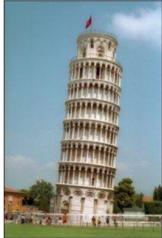
Leaning tower of Pisa, Italy
