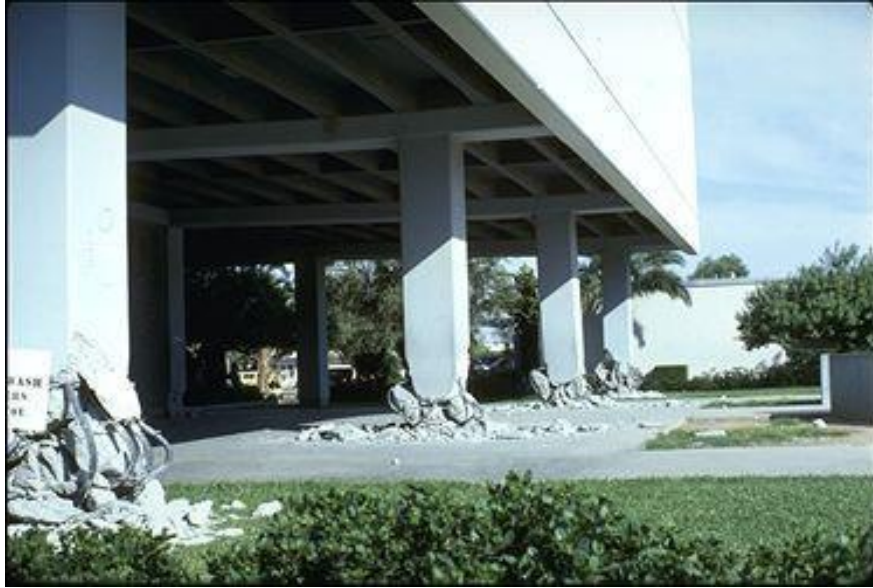
Crushing failure – 1985 Mexico earthquake.
