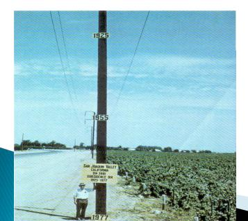
Subsidence of the land surface caused by the extraction of ground water, near Mendota, San Joaquin Valley, CA. Signs on the pole indicate the positions of the land surface in 1925, 1955, and 1977. The land sank 30 feet in 52 years.
