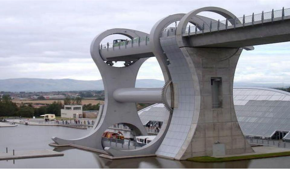
Closing the gate , regulation of level of water and "tubs" rotation takes 15 min. only.
