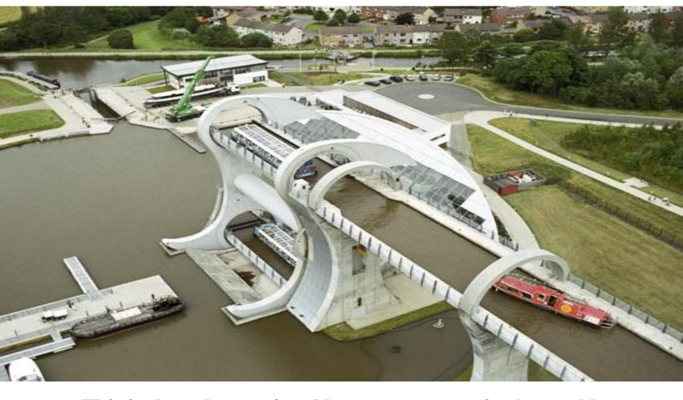
This is the only rotational boat transporter in the world. It has two arms and each arm forms a kind of huge tub filled with water. Boats enter the table then the tub locks up and the huge arm starts
