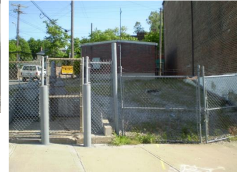
Pipelines for natural gas & other chemicals
