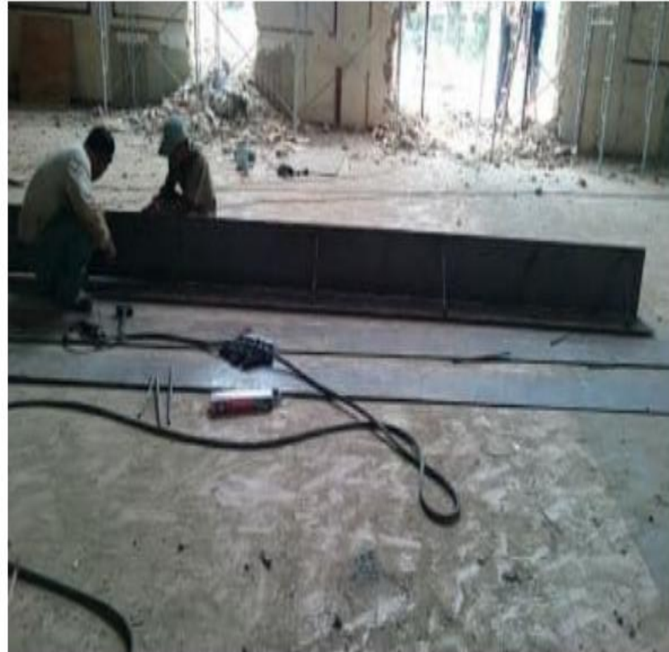
Fig. 4: Welding steel jacket
