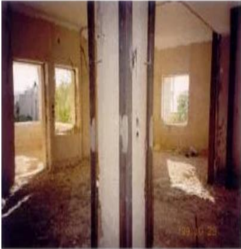
Fig. 3: Column strengthened with steel angles
