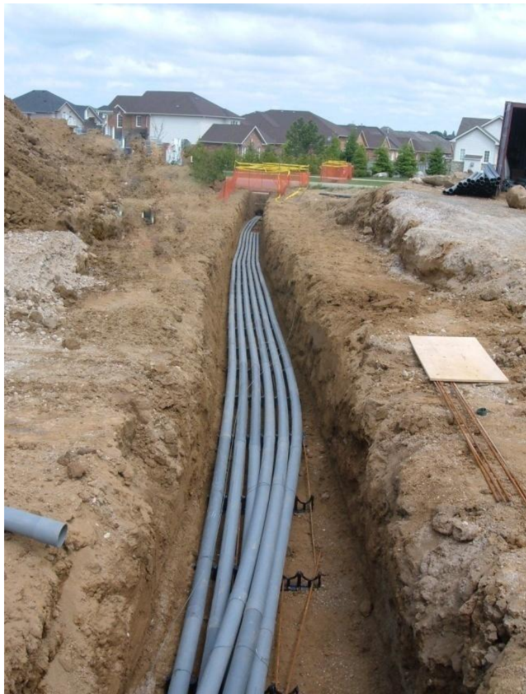
Fig.8: Cable Direct Laying
