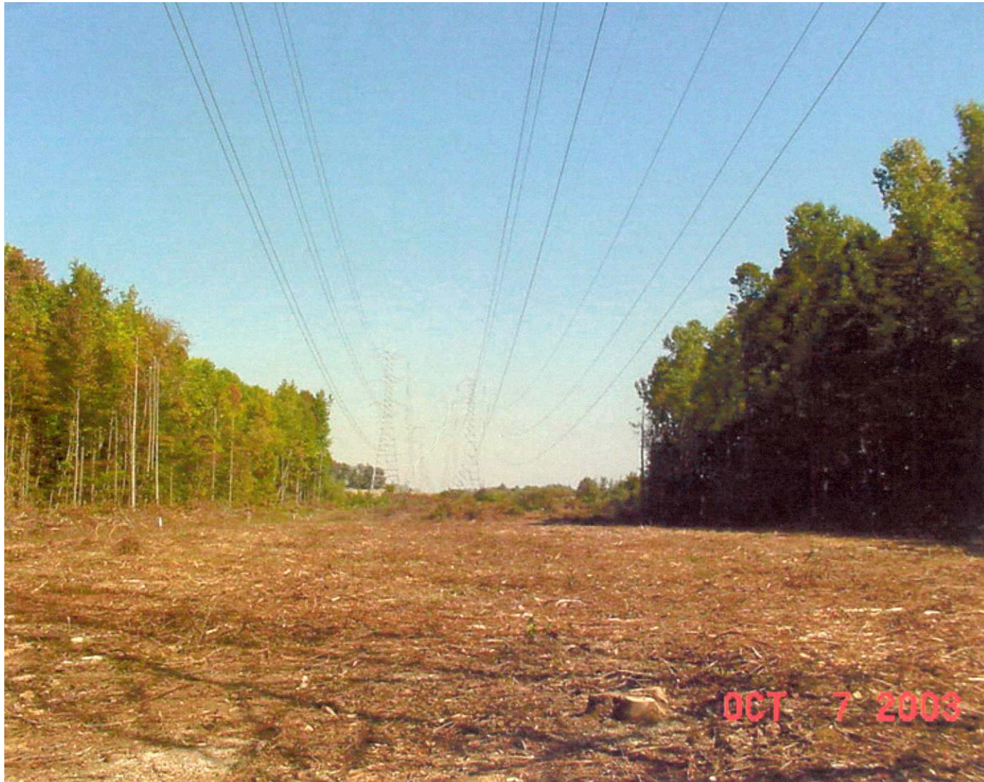
Fig.10: Transmission Line after Tree Trimming
