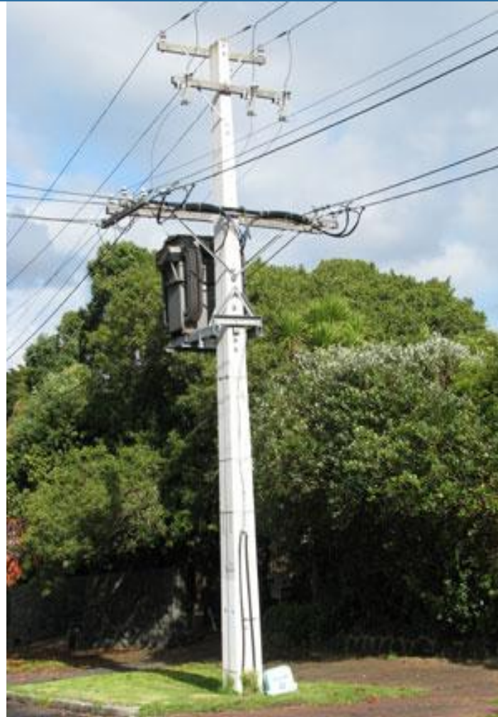
Fig: Reinforced Concrete Poles
