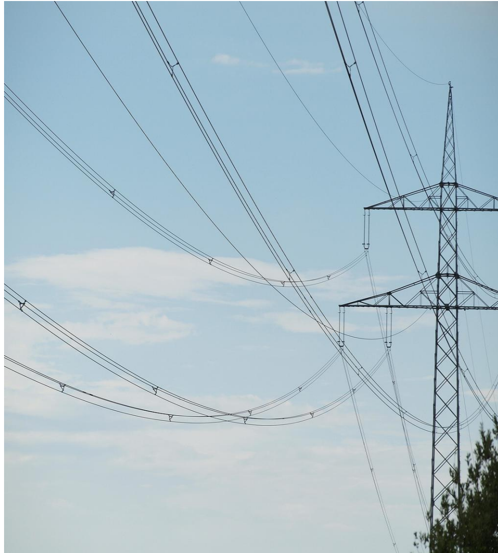
Fig: Bundled Conductor
