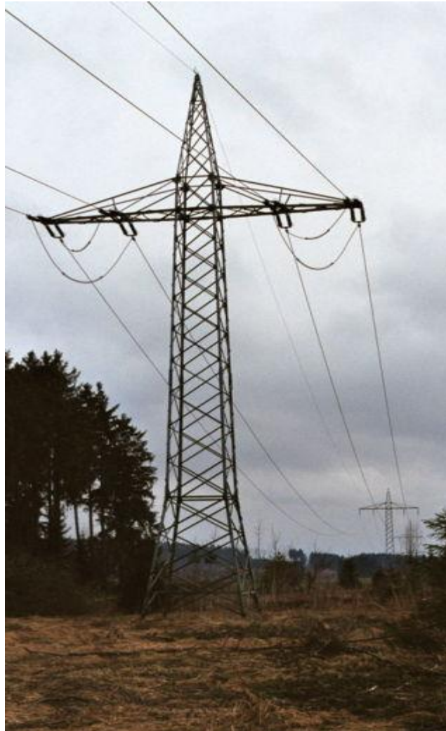
Fig: Tension Tower
