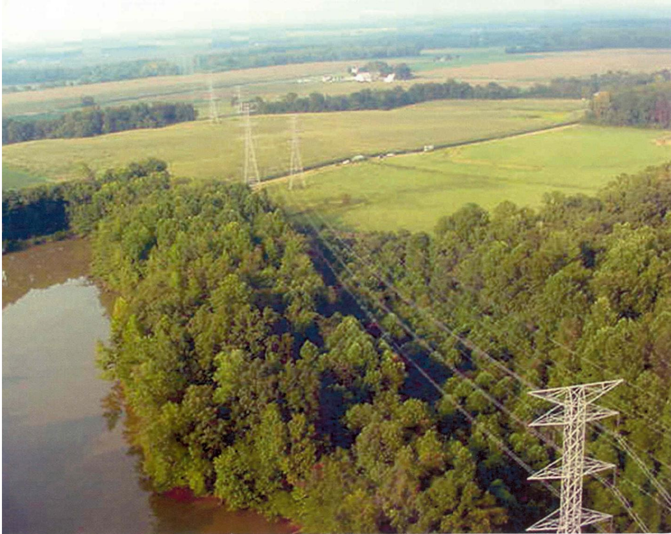
Fig.9: Transmission Line Before Tree Trimming
