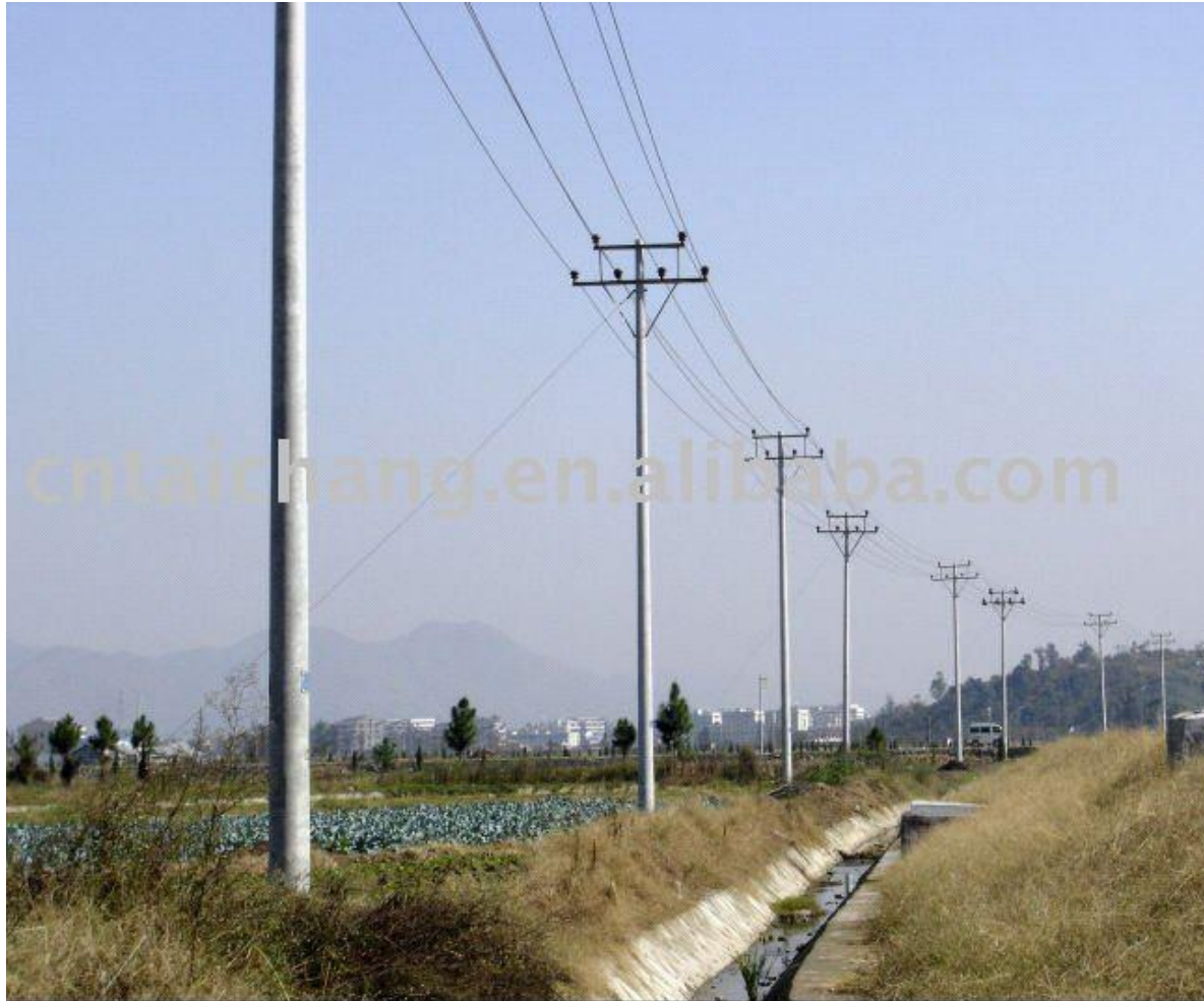
Fig: Reinforced Concrete Poles
