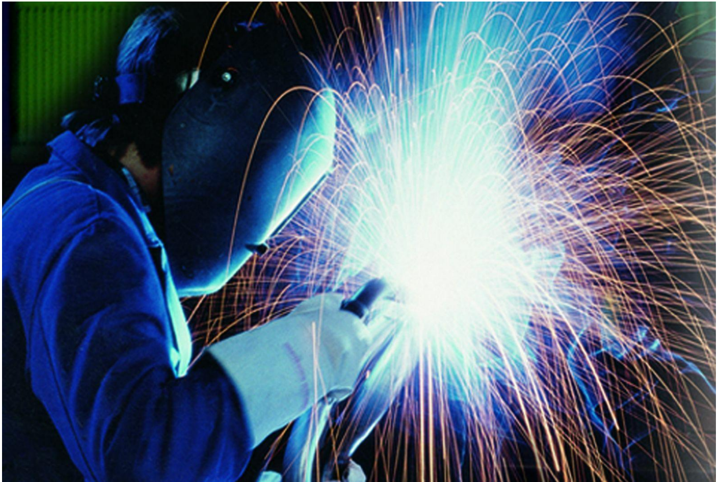
FIGURE – Welding operation
