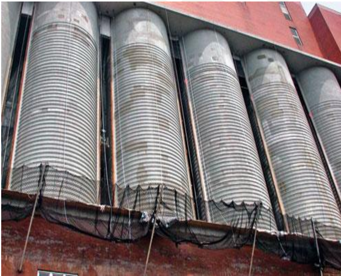
Figure: External prestressing in circular tanks
