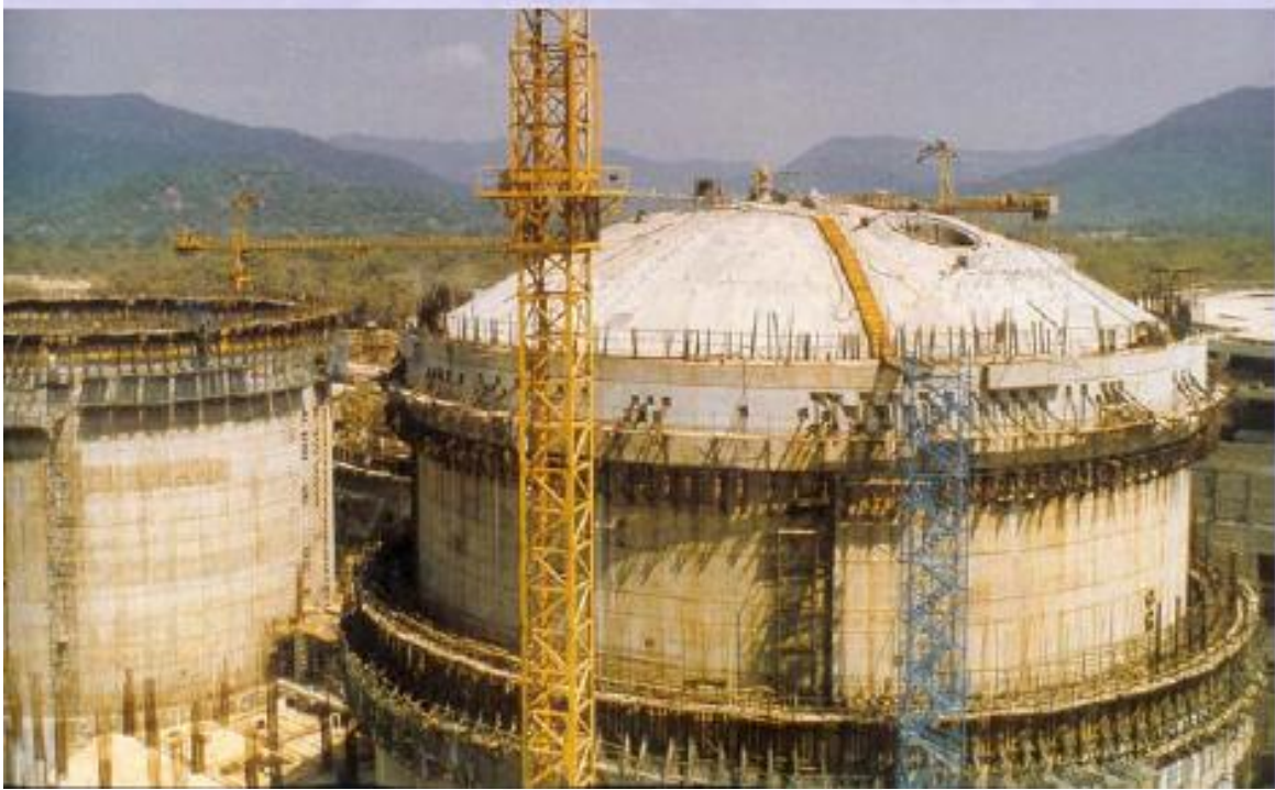
Figure: pre stressing of circular tank
