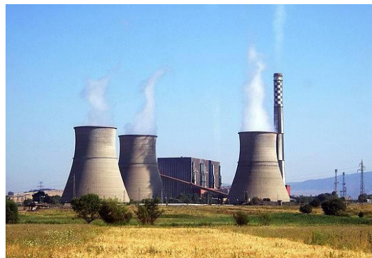
Figure: Cooling Tower
